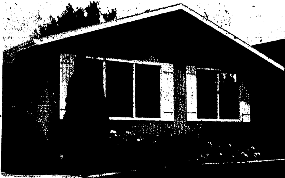
Before the Retrofit: R-8 walls Double glazing R-15 ceilings Yearly electrical usage: 40,662 kWh
