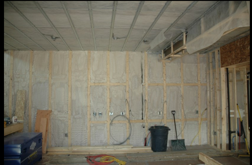
Foam insulation at party wall
