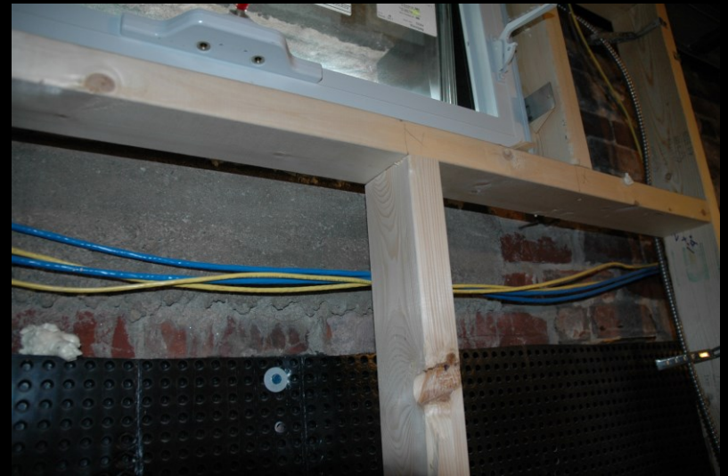
Gap between framing and exterior masonry wall to eliminate thermal bridging
