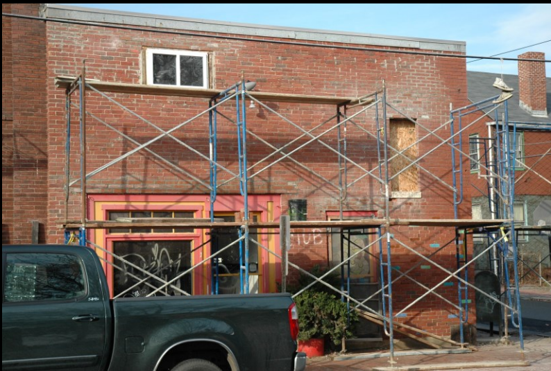
Repointing - Existing window not removed, yet
