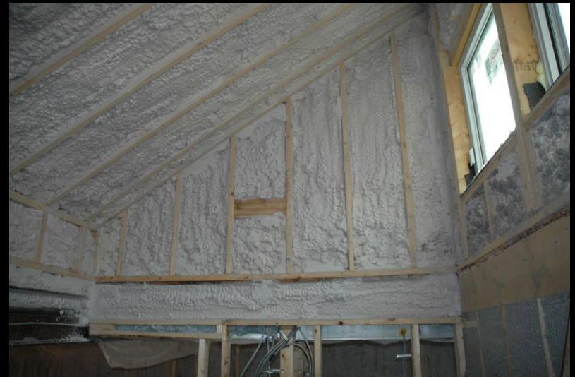
Foam insulation at roof monitor
