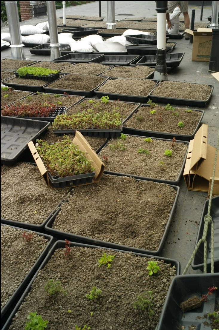
Installation of vegetated roof
