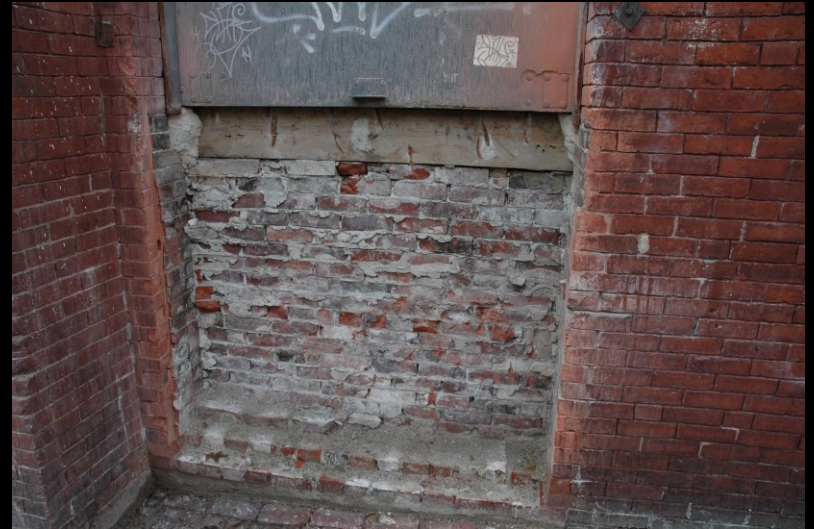
Demolition - Removing brick to create loft entry
