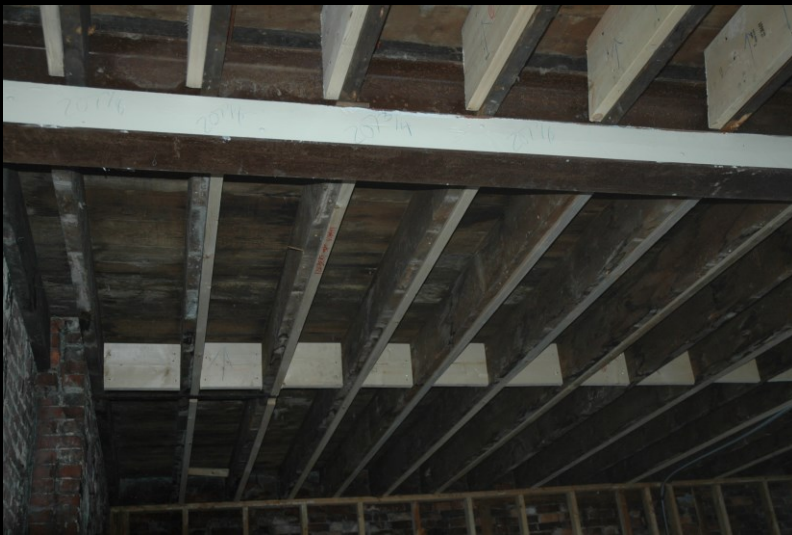
Reinforced roof structure
