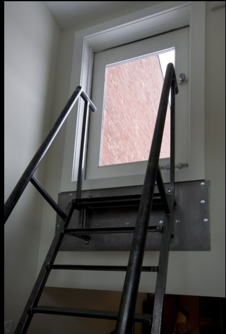
Folding stair to roof deck
