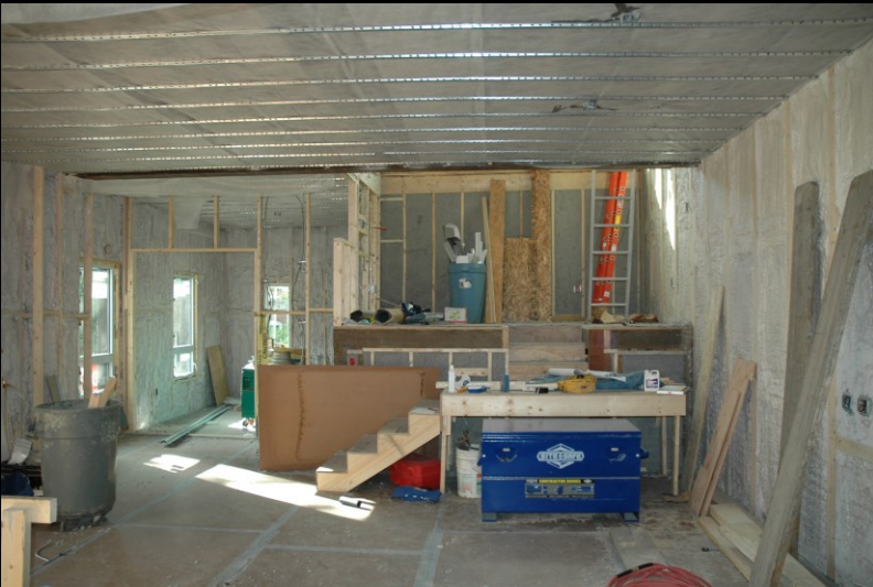
Insulation - Foam in walls; foam+cellulose in roof
