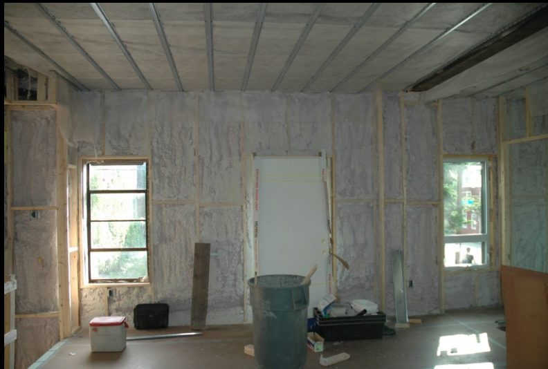
Foam insulation at exterior wall
