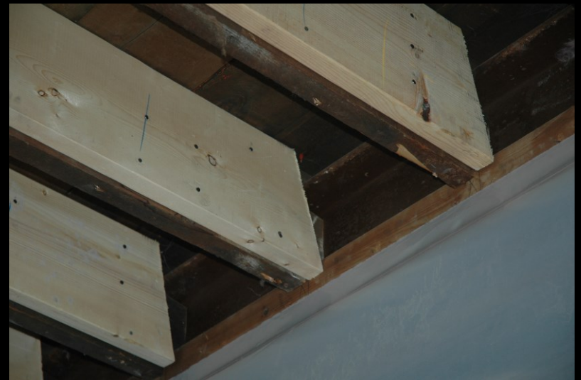
Detail of roof reinforcing
