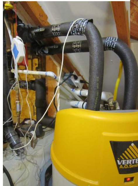
First Co hydronic air handler with ECM motor and low total external static pressure, paired with a condensing tank water heater rated at 97% efficient.
