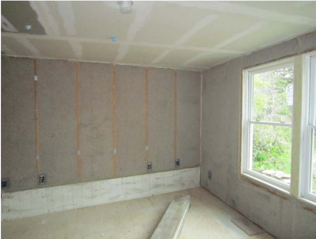
Wall spray Cellulose application
