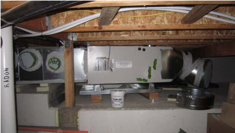
First Co hydronic air handler with ECM motor and low total external static pressure, paired with a condensing tank water heater rated at 97% efficient.
