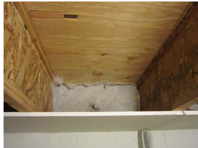
Cellulose behind netting at rim joists
