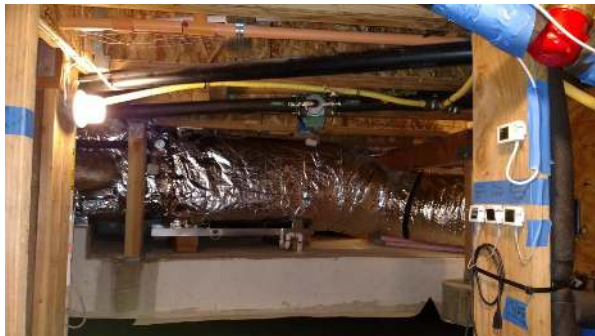
First Co hydronic air handler with ECM motor and low total external static pressure, paired with a condensing tank water heater rated at 97% efficient.
