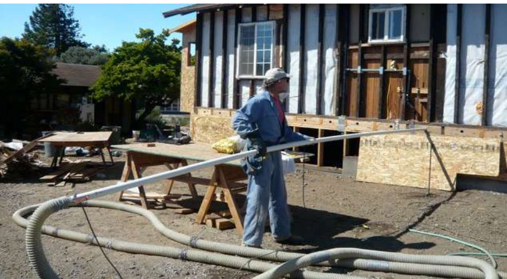
Crawlspace R41 insulation in floor
