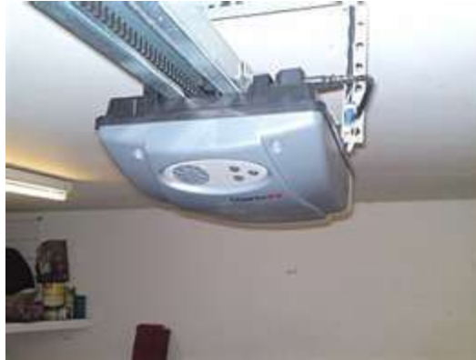
Add switch leg to garage door operator
